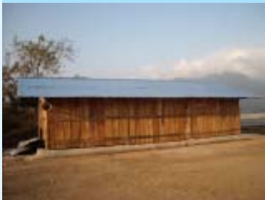
LUTHA CHURCH OF CHRIST, ONE OF THE SEVEN NEW CHURCHES PROVIDED ZINC ROOFING BY IDES
